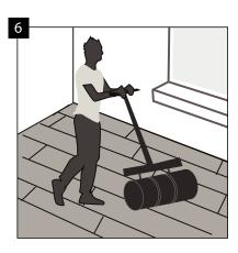
Not later than 60 minutes after gluing the panels, use a 50 kg roller in order to press the glued panels to the substrate accurately and evenly.
