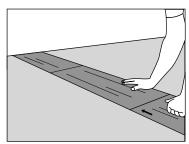
**2.** Lay the panels without stress and adjoining each other. When laying large tiles, follow the direction of the arrows on the back.
